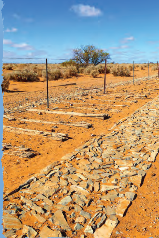
A section of the hand laid stones. ▲
